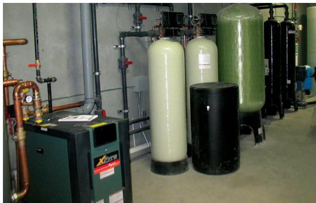
A volume water heater, water softener, carbon filter and flow tanks complete the water treatment for all chemical application and fresh water rinsing.
