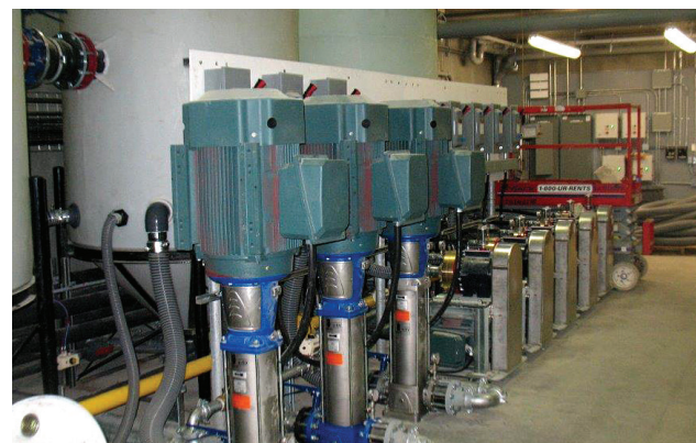
Three high-volume pumps provide water to various wash function in the wash process. In the background, five high-pressure pumps apply a final fresh water rinse.
