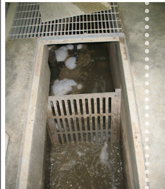
▼ Water passing through a bar screen.
